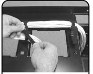
Route cable onto tray and fasten with hook and loop managers. Tray allows routing of cable along three separate horizontal pathways via three rows of hook and loop managers. Cable bundles can then be routed down the middle and/or sides of tray (as shown).
