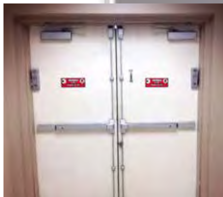
Multiple door monitoring with built-in external reed switches, too.
