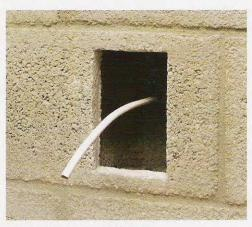
For masonry construction... Make hole in block. Pull wiring through plastic block bushing and opening in block.
