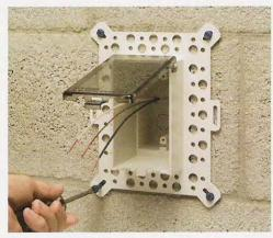
Attach Recessed IN BOX to masonry block. The holes in the flange are designed to allow stucco to bond to the substrate.
