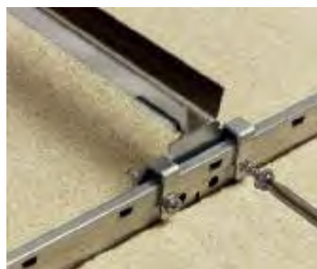
5 Option Use sheet metal screws – where required by local code – to hold ends securely on grid (screws not included).
