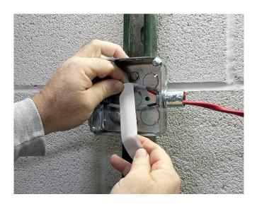
7. Reposition spliced leads to insure they are in line with cables as illustrated, and apply UL Certified fire-rated putty (firestop) to cable entrance and exit box fittings.
