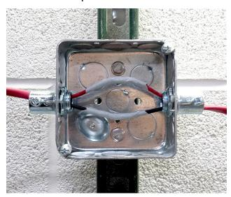
6. Apply 10" of fiberglass tape, using ½ lap overlay, to complete splice coverage of each lead termination in order to have two layers of tape coverage.
