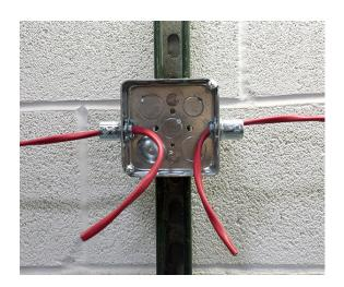
2. Carefully strip approximately 3" of outer jacket to expose insulated leads.
